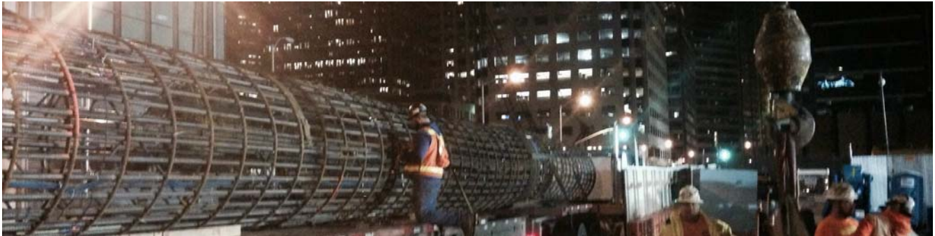
The Lower Rebar Cage Arrives on the Job Site
