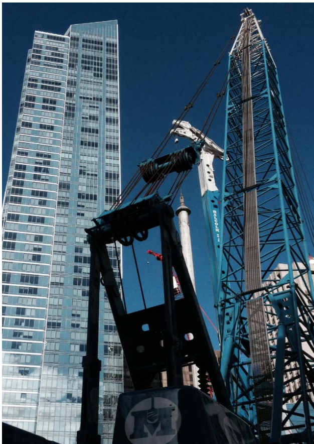
Drilling the Test Shaft
